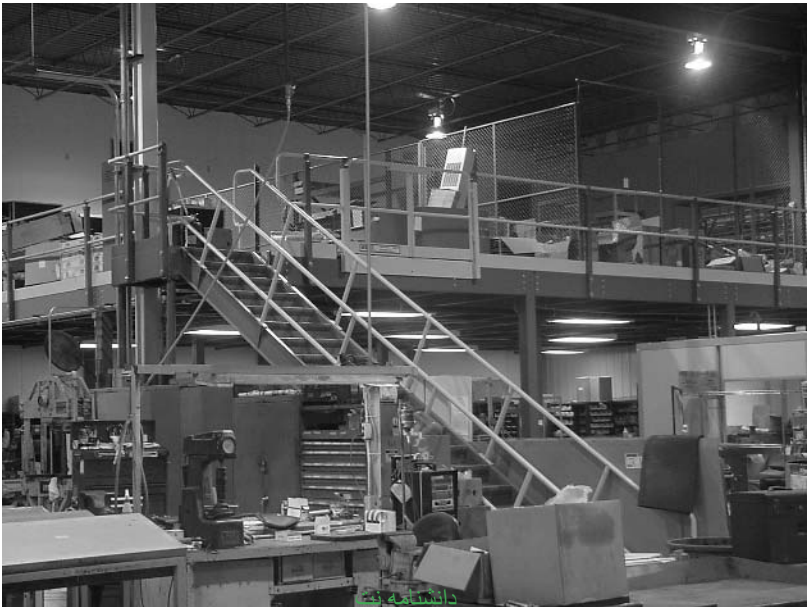
Figure 7-3. A mezzanine can be installed to provide additional parts storage space.
